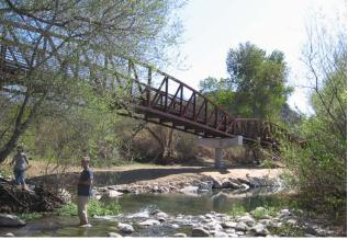
A beautiful bridge for pedestrians and bicyclists using the Ojai Valley Bike Trail was installed in 2012 at the very end of San Antonio Creek, just before it merges with the Ventura River. The bridge replaced an old concrete crossing over some box culverts that frequently became plugged with woody debris during storms.
