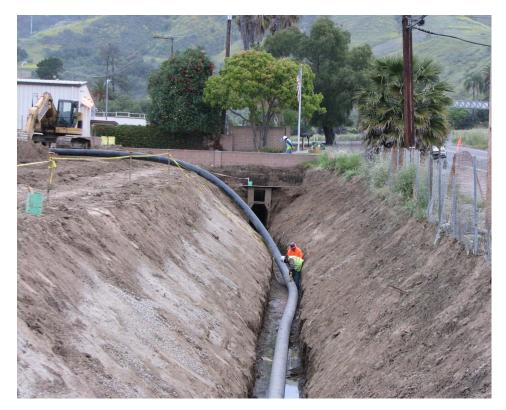
Ojai Valley Sanitary District replaced and relocated an 800-foot section of underground sewer pipe that ran along the edge of San Antonio Creek. This pipe was vulnerable to damage during floods, which could lead to sewage spills. The district also completed a \$6.5 million Ventura Avenue Sewer Improvement Project (photo above) to update aging infrastructure and reduce energy demand. Photo courtesy of Ojai Valley Sanitary District.
