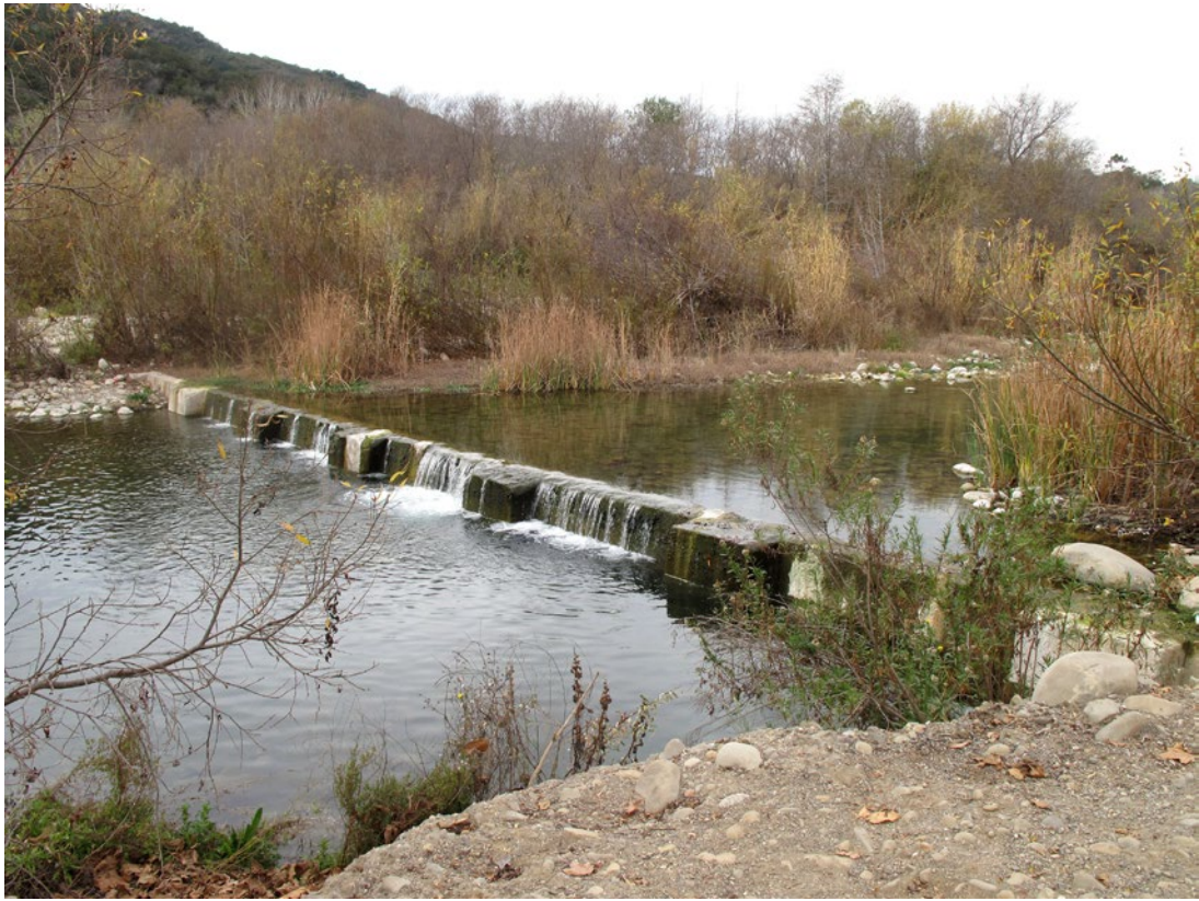
City of Ventura's Subsurface Diversion Structure at Foster Park. The diversion dam slows the flow of subsurface water downstream. The City of Ventura extracts water at the structure and also has a number of wells just upstream.
