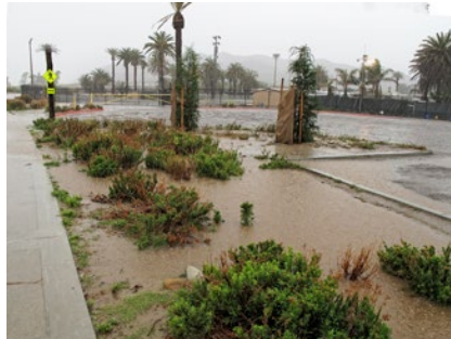
Bioswale, Surfers' Point, Ventura
