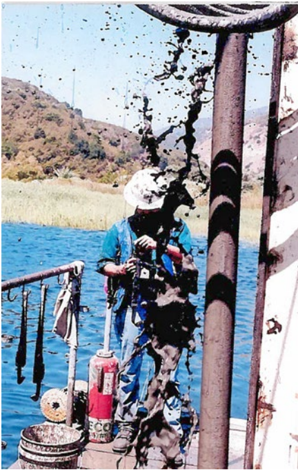
Methane Gas Eruption During Drilling, 2001. During sampling, some drill holes encountered methane gas pockets below the water, which caused sediment "geysers" and turbulent boils in the water. The methane is produced by rotting vegetation.
