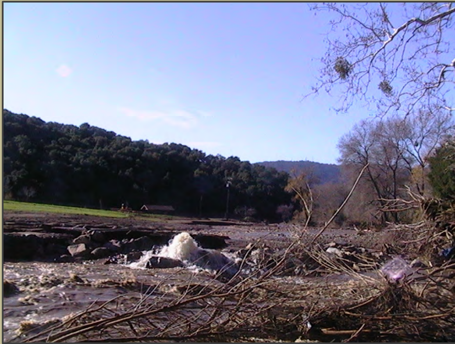
Sewer overflowing in San Antonio Creek, 2005 (Photo: Ojai Valley Sanitary District)
