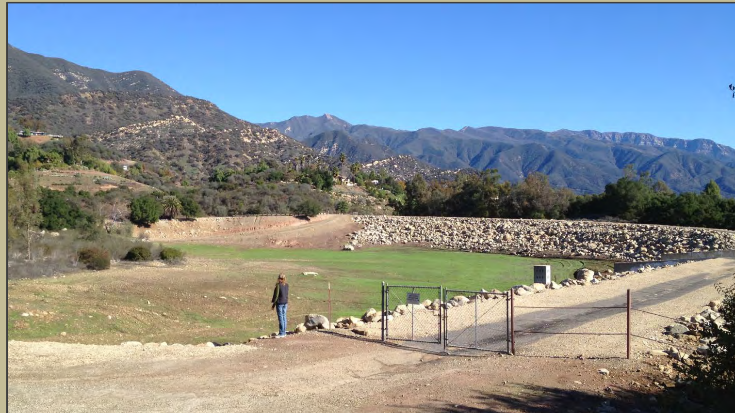
Stewart Canyon Debris Basin, Ojai 10 acres in size, 328,300 cy capacity (Photo: Lisa Brenneis)
