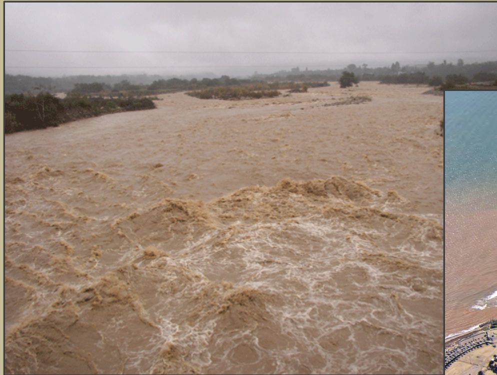
Upstream of Hwy 150 Bridge, Ventura River, 2005 (Photo: Copyright David L. Magney)
