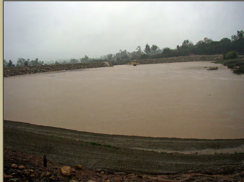
Stewart Canyon Debris Basin full, 2005
