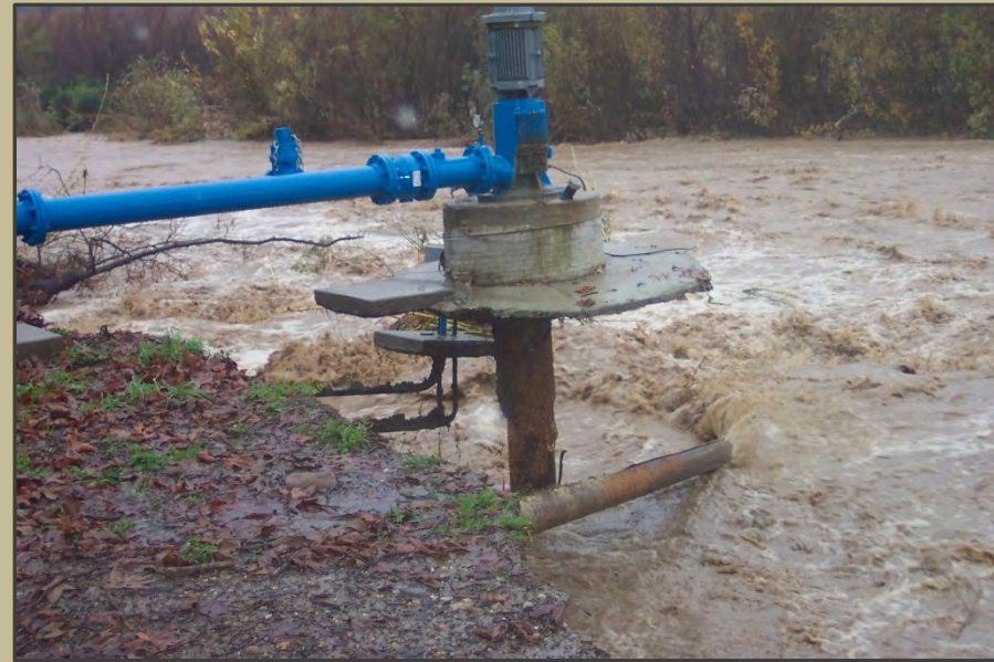
City of Ventura's Nye Well 1A, Jan. 2005, which replaced Nye 1 lost in a previous flood. The Feb. 2005 flood took out the rest of the well.
