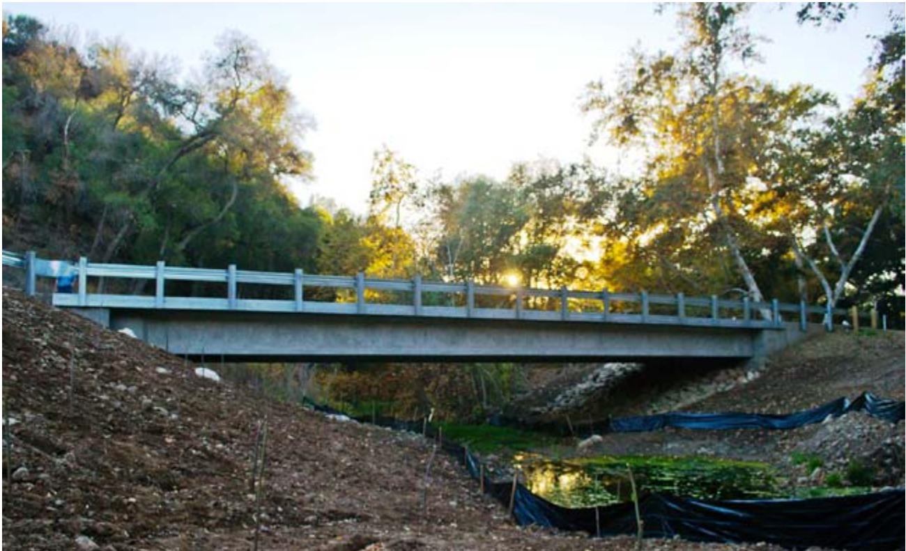
A clear span bridge was constructed in 2013 on San Antonio Creek near the confluence with Stewart Canyon Creek, just south of the City of Ojai. The bridge replaced a fair weather crossing on private property. Photo courtesy of Bill O'Brien.
