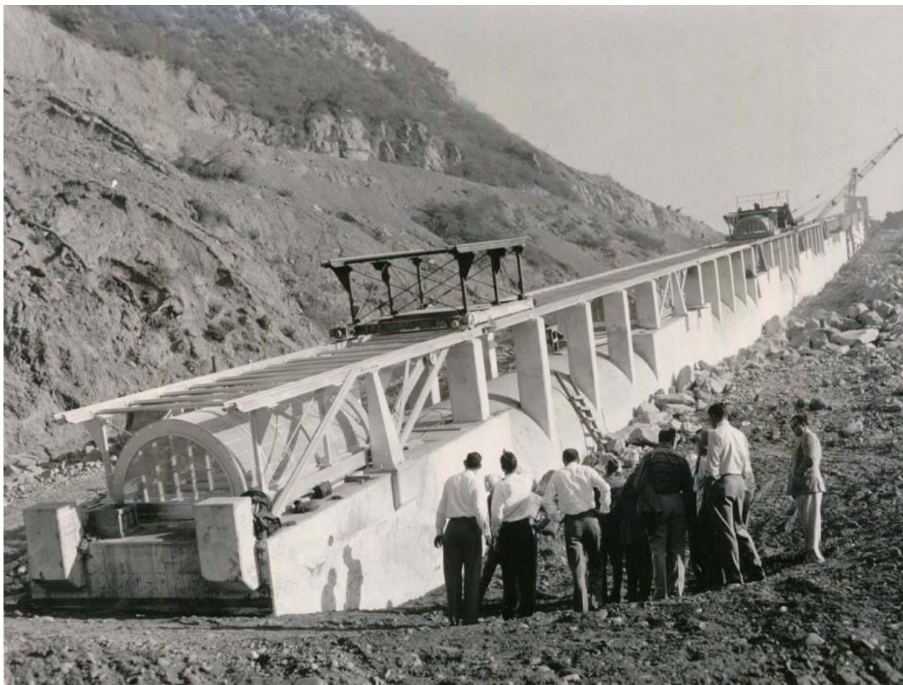
Lake Casitas intake structure under construction, December 1958. The intake structure is on the reservoir side of the dam, and moves water from the reservoir to the treatment plant.
