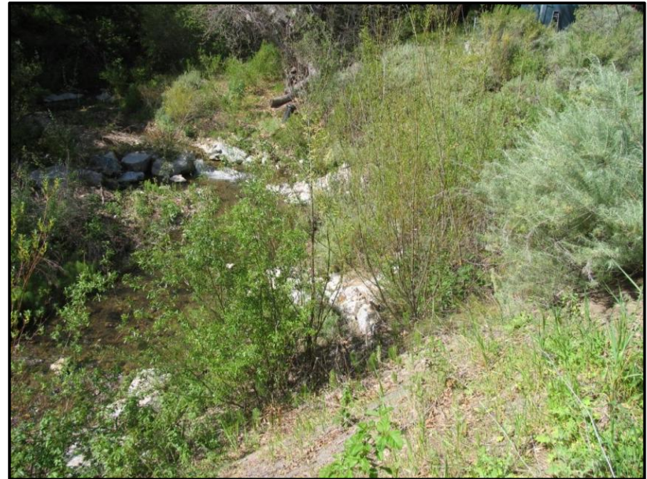
Soil Wraps with Rock Toe Protection
