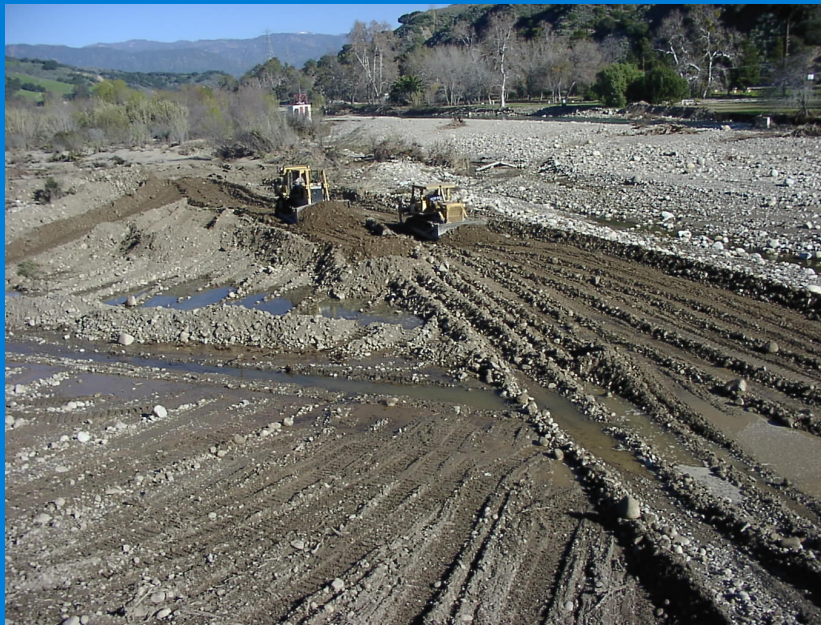
Ventura River Channel Modification
